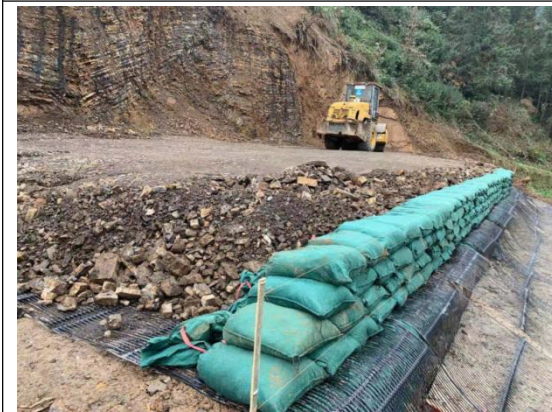
袋装土临时拦挡
